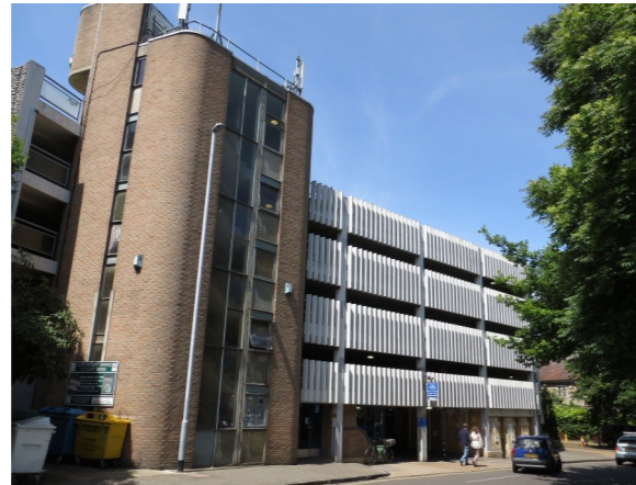
Photograph of existing car park
